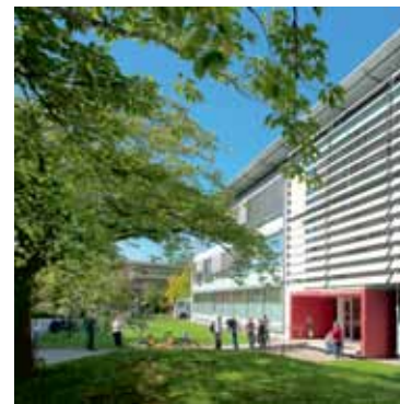
The Otto-Meyerhof-Zentrum on the Medical Campus of the University of Heidelberg
