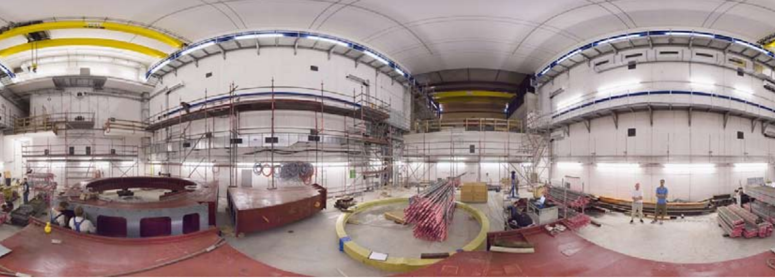
Gantry Raum Before Gantry assembly
