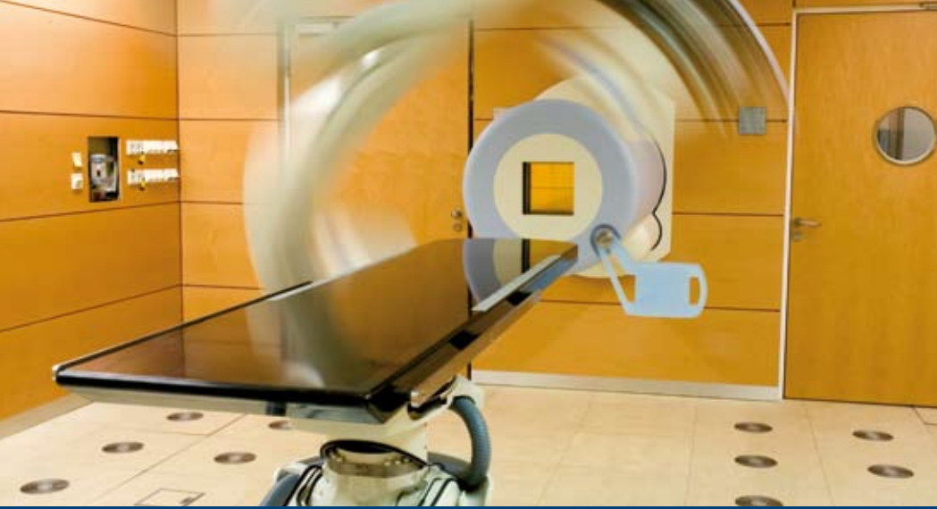
HIT treatment room with rotating X-ray systems
